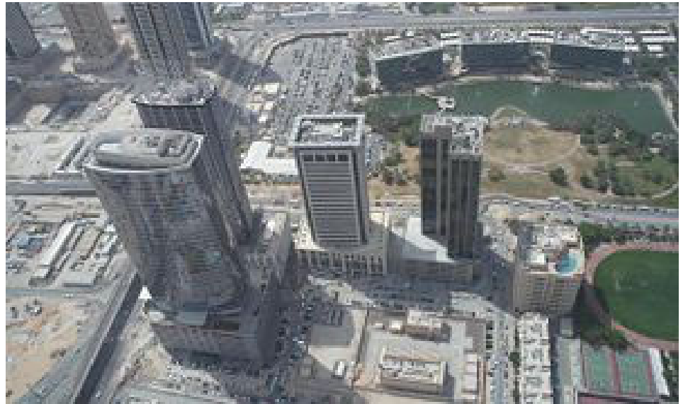
Buildings under construction in the Dubai Media City Complex (image courtesy of Dubai Media City)
